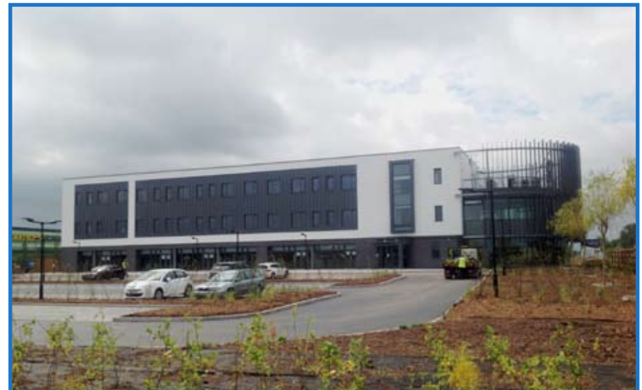
Bridgwater Enterprise and Innovation Centre
